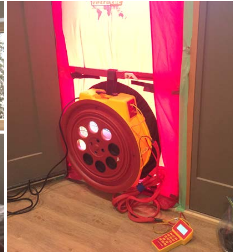
Right: Blower door testing during a builders' workshop held in Invermere; the home is expected to exceed EnerGuide84 (equivalent to Part 9, Step 3).
